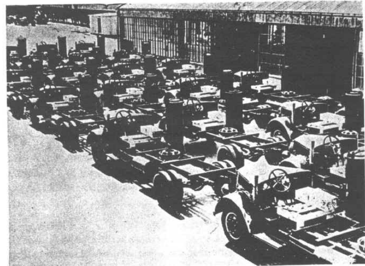
Germany, about 1943. Mass production of gas producer vehicles, Imbert factory, where some 500,000 gas producers were manufactured during World War II. (E. E. Donath)
